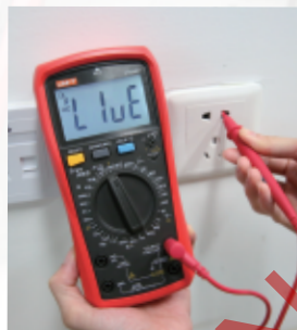
Live and nature wires identification
