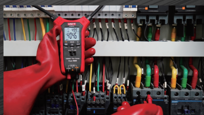
AC voltage test in the power distribution box
