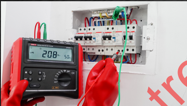
💡 AC voltage test
