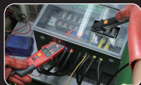
Phase rotation test
