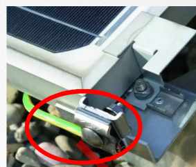
Poor grounding
