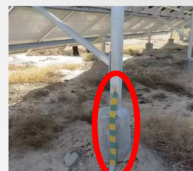
Poor grounding
